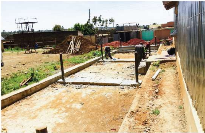
Foundation Preparation
