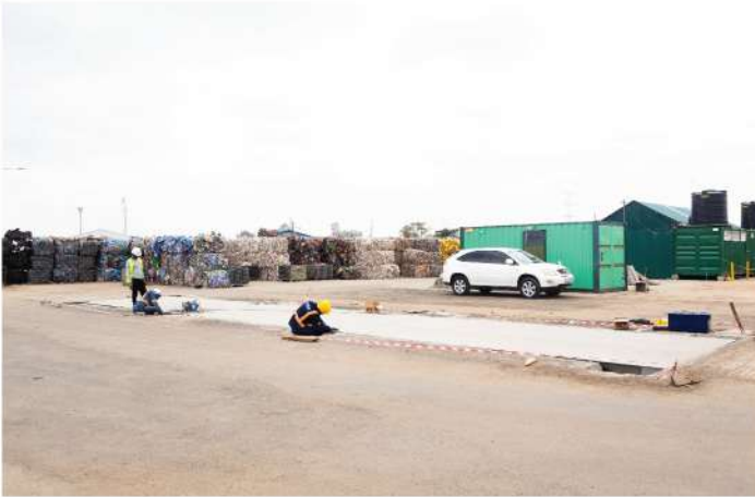
Installation of decks and loadcells
